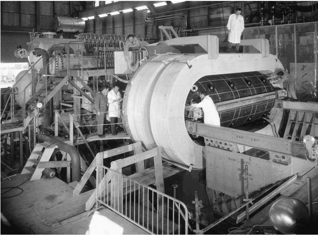
Figure 1: The body of Gargamelle is inserted into the magnet coils.
