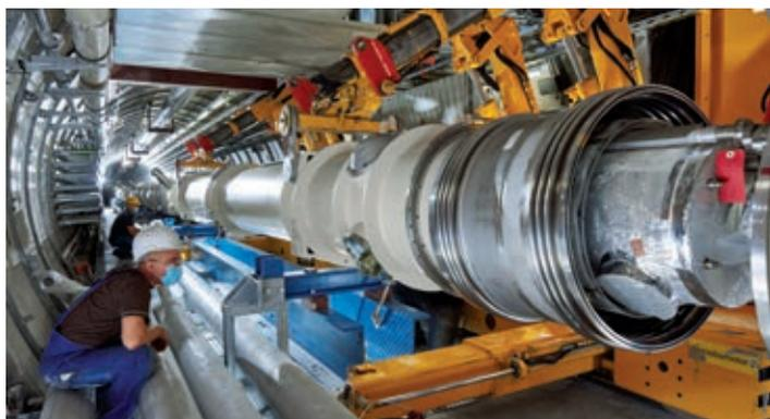
Installation of one of the last superconducting magnets for ALPS II
