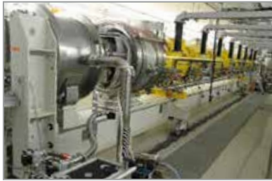
Figure 2 Cryomodule mounted on the test stand with RF power couplers connected to the waveguide distribution, ready for closing the cryogenic connection
