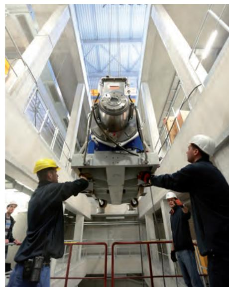
Workers guide the injector klystron into place using a crane in the injector hall at European XFEL's Bahrenfeld site.
