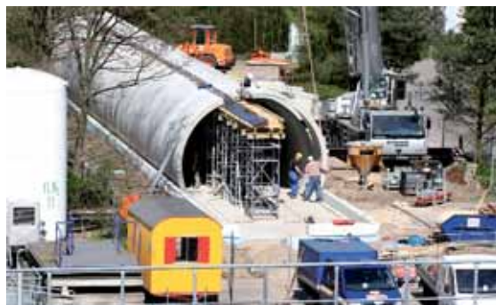
The XFEL tunnel model is assembled from concrete elements in the finest April weather. Only the 64-m-long sheet metal building is now missing.
