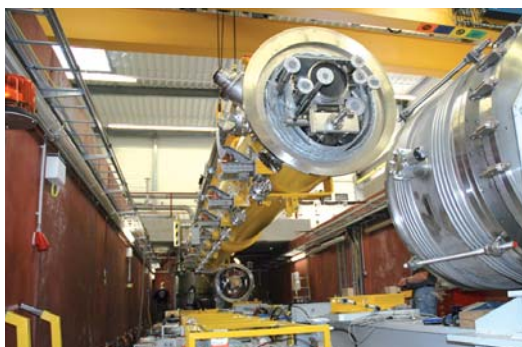
Module 6 in the new test stand. Soon it will be installed in the FLASH linac—an important step towards the wavelength design value of 6 nanometers.
