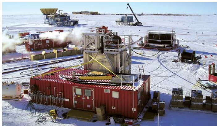
In front you see the red IceCube drilling and installation container, in the background the steaming flow heater for the drilling water.
