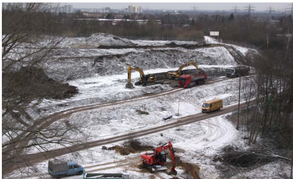
View of the construction site DESY-Bahrenfeld behind Building 2, where the soil of part of the Lise Meitner park is being removed.
