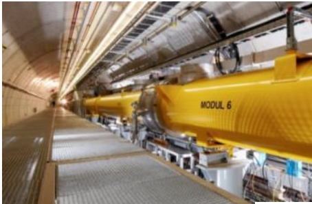
> TESLA type superconducting accelerating modules 1.3 GHz
