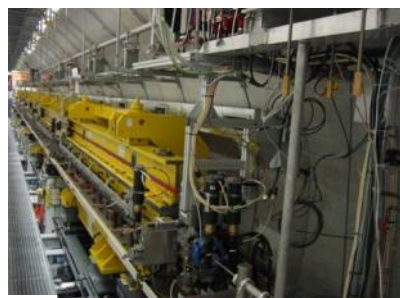
> FLASH1 fixed gap undulators
