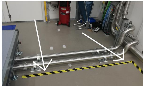
**Figure 2.19:** Pipe anchors with the seismometer positions pointed out.
