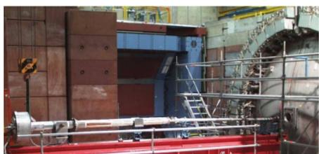
The **superconducting magnet GO** and the central beam pipe are prepared for installation in the liquid argon cryostat. The GO magnet provides vertical focusing and an 8 mrad bend for the electron beam in a compact coil design.
