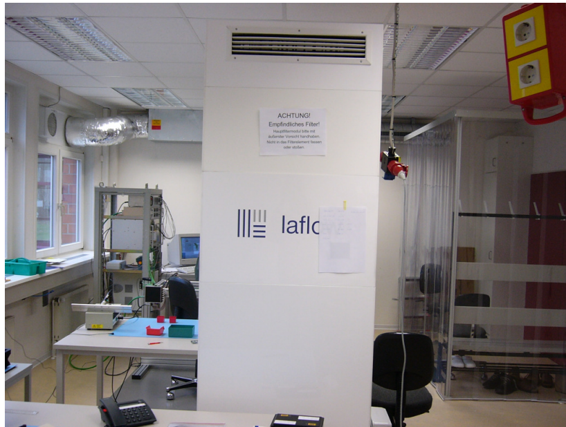
Grey room with air filter unit and humidity control in Hamburg.
