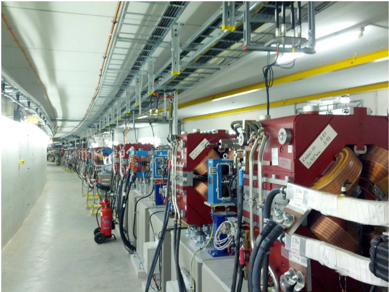
Figure 4: PETRA III extension North. The new DBA like lattice of the extension section North is shown in the photo from April 2015.
