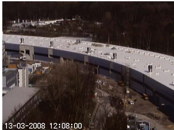
Figure 2: The new experimental hall of PETRA III. The photo shows the construction site from inside the ring. This photo is taken from the webcam: http://petra3.desy.de/webcam .
