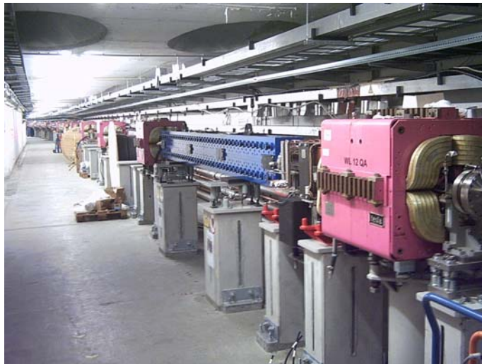
Figure 4: One wiggler cell in the PETRA III tunnel. The synchrotron light absorbers are installed downstream of the wiggler and in front of the quadrupole magnet (WL 12 QA).
