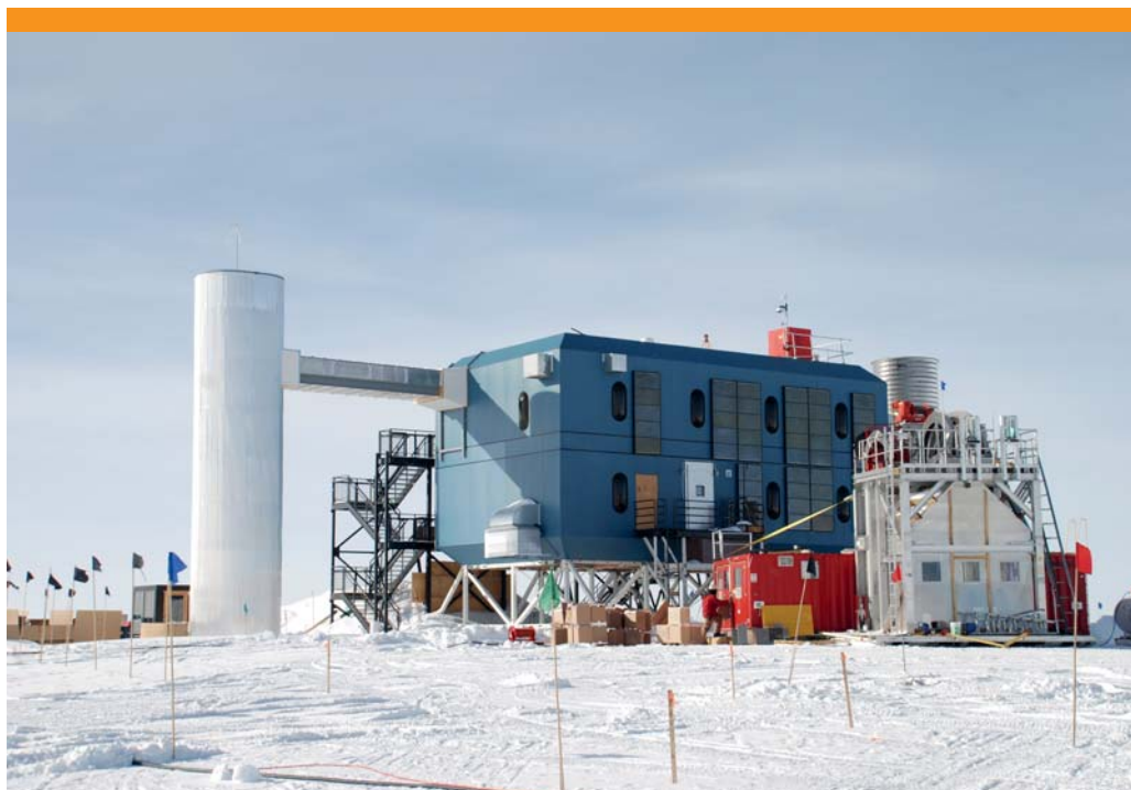
The hot water drilling facility (on the right) is drilling the hole in front of the blue "IceCube Counting House" where all IceCube data are collected.
