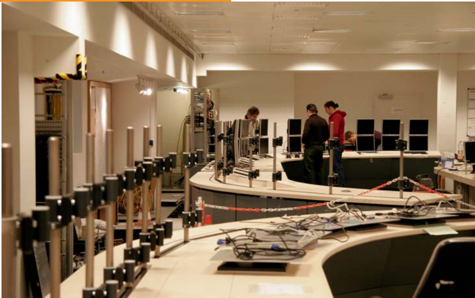
Almost completed: the new control desks are already installed but are still to be connected.
