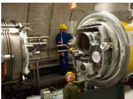
The seventh accelerator module is installed in the FLASH tunnel.
