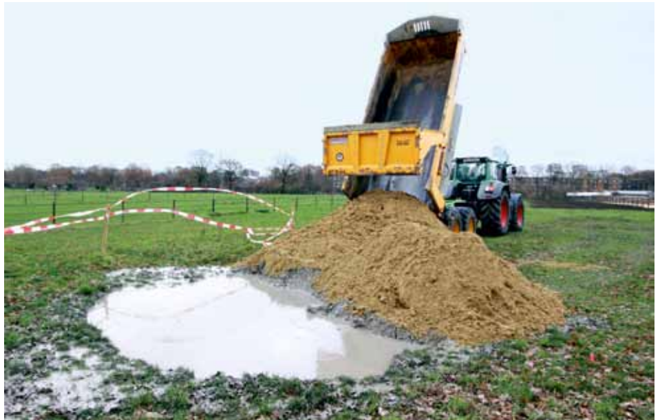
Two days after the subsidence occurred on the horses' pasture, it was filled with sand.
