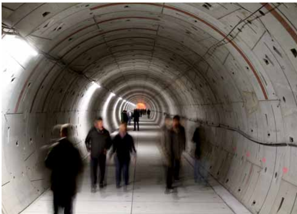
In 2013, the first accelerator modules will be installed here: the European XFEL tunnel construction has now been completed (Photo: M. Mayer)
