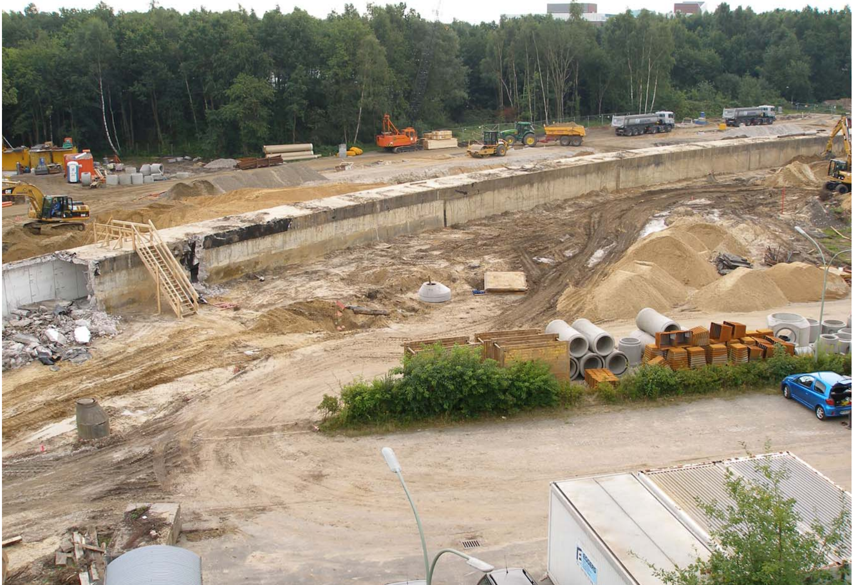
PETRA III construction site, 2.8.2007, 9:52
