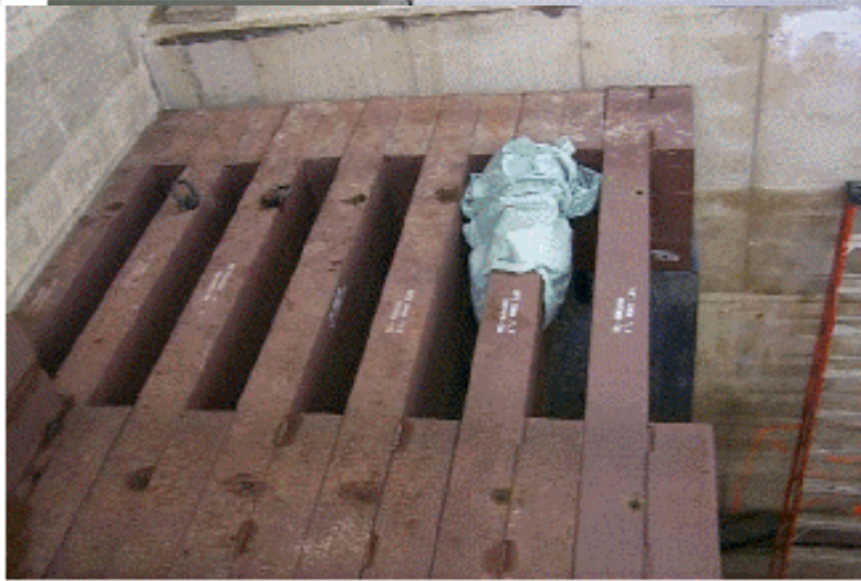
Steel installed in the Target Pit
