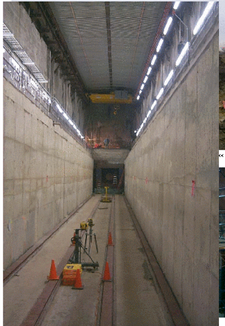
Target pit with installed steel in center of phase
